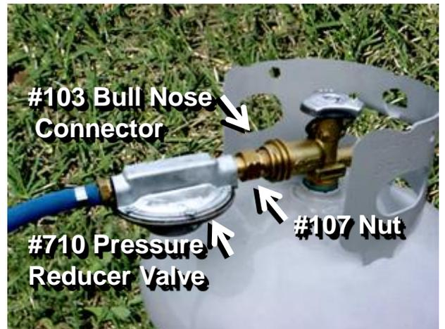
Tighten nut #107 with a wrench.
